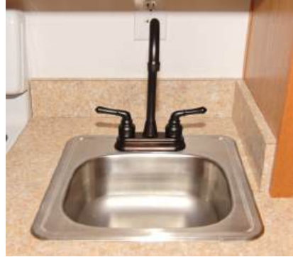
Wet Bar Sink
