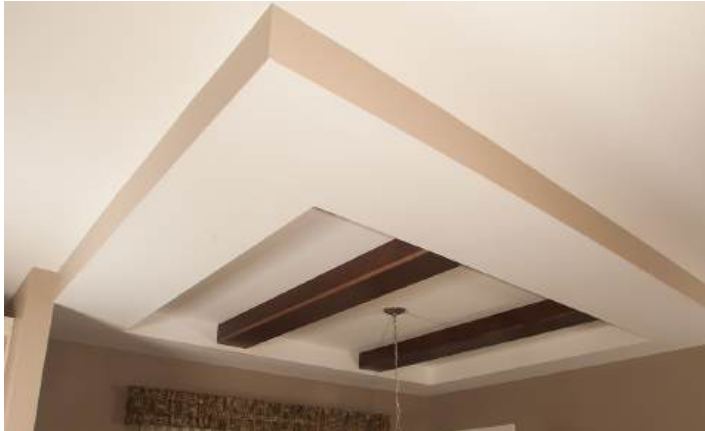
Tray Ceiling with Wood Beams
