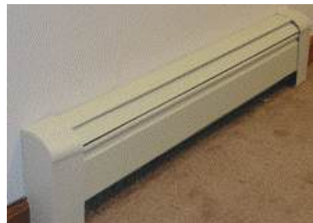
Hot Water Baseboard Register
